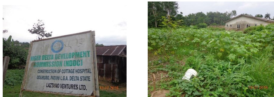
Plate 4.6a: Uncompleted cottage hospital at Odorubu community
