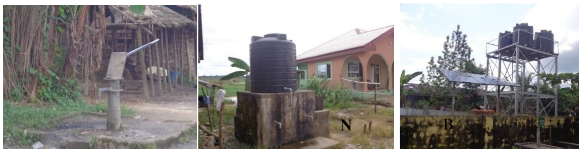
A: Manual Borehole Pump B: Private owned Borehole C: MDG water project
