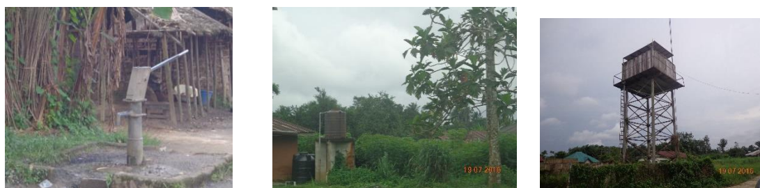
Plate 4.6d: The various water facilities in the two communities: A hand-pump provided by the government, a private borehole and articulated, but non-functional water facility
