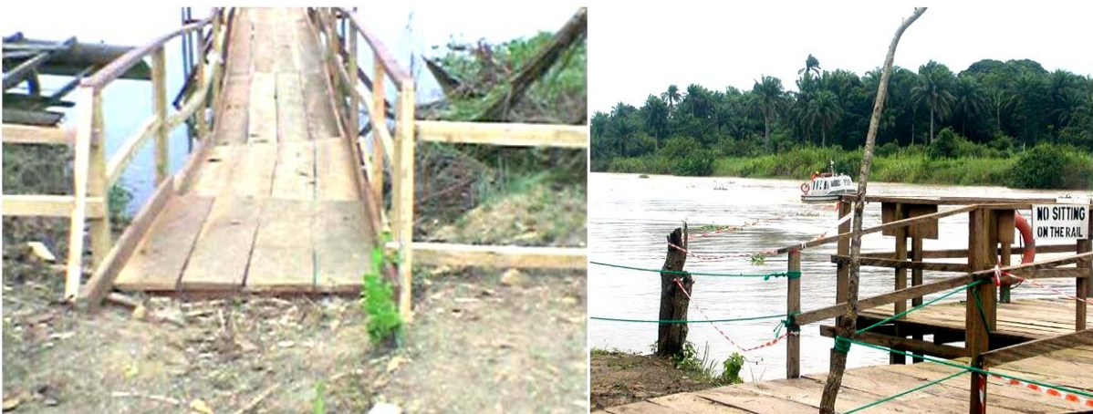
Plates 3.2: Examples of improvised Jetties for the purpose of workmen boat embarkation and disembarkation for water borne activities
