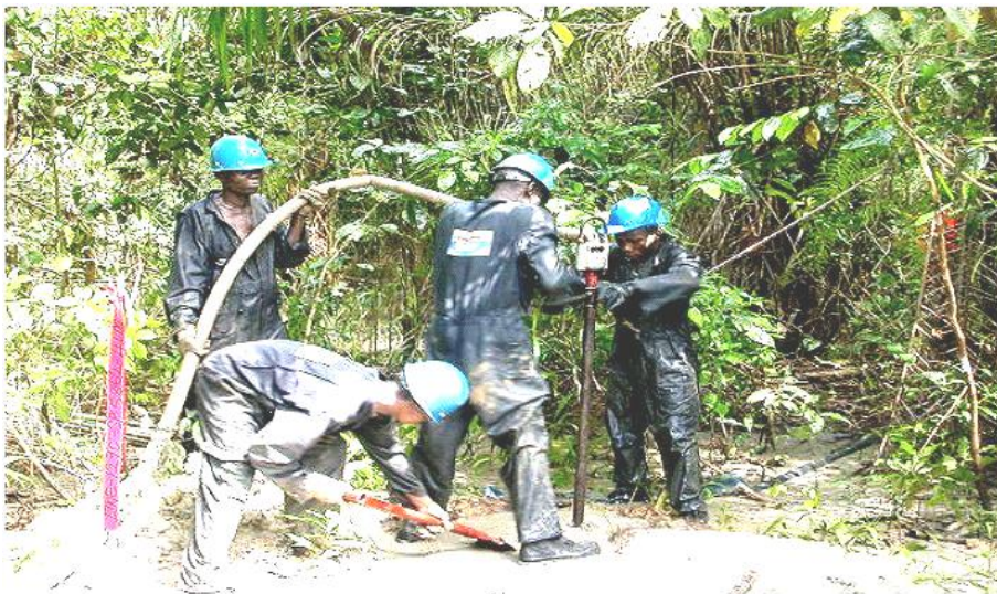
Plate 3.8: A typical Single deep hole SDH rotary flushing method
