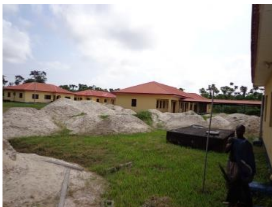
Fig. 4.6k: Cottage hospital in Ogidigben being renovated
