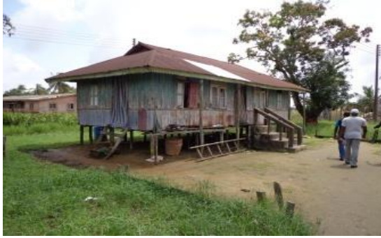
Plate 4.6f: Several houses in the host communities were raised to avoid the seasonal flood
