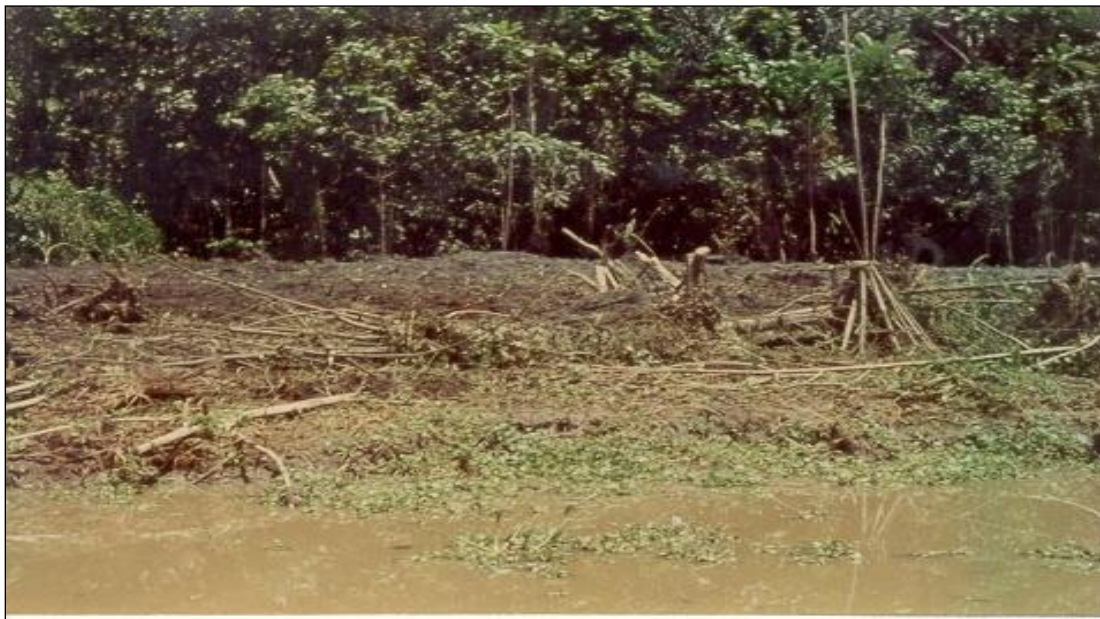
Plate 5.1: Bush cleared area prior to dredging in Opukushi field (Macgill, 1996). Observe the impact on water: Turbidity, Suspended solids
