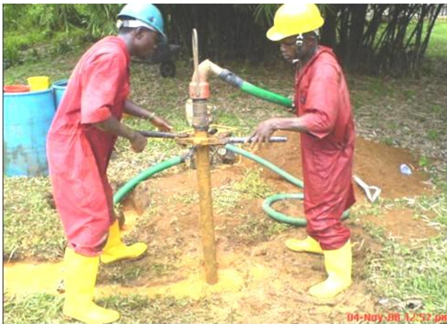
Plate C: One of the boreholes being drilled
