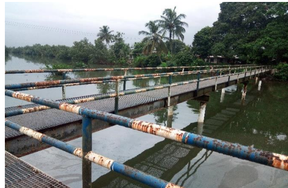
Iron Jetty at Nkpokiri
